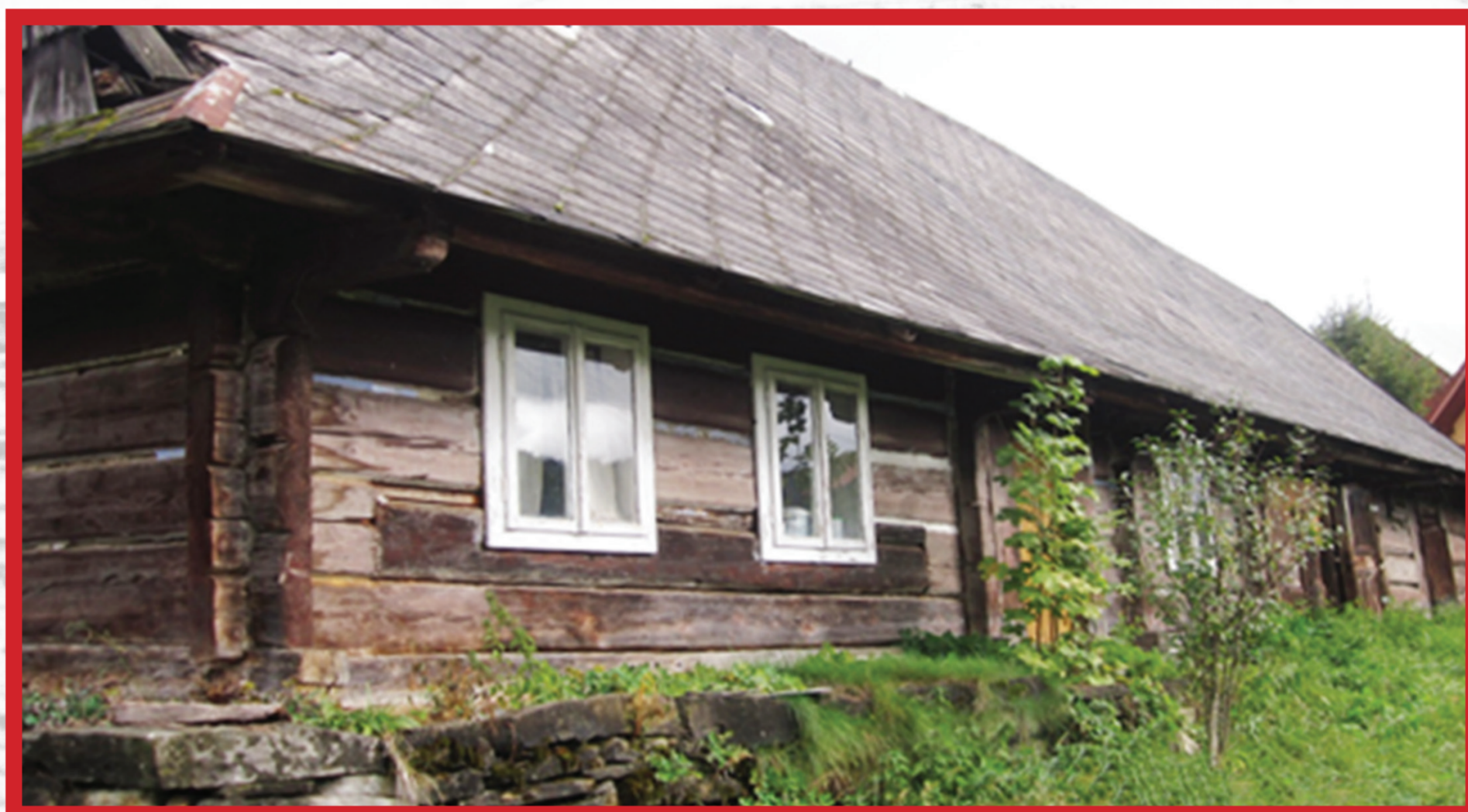
The cottage in its current condition
