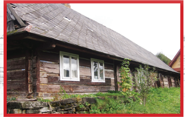
The cottage in its current condition
